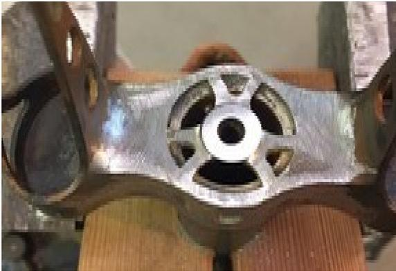
**Photo 2:** A fender mounting boss that would provide access, if a bit fiddly, for removal of the wooden plug used with the Herse method.
