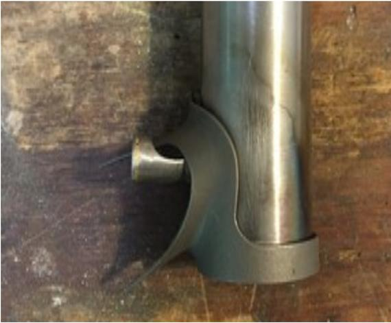
**Photo 8:** Lug being installed by nesting the upper point in the sculpted portion of the capsule receptacle. The lug reinforcing ring is about to be pushed to the left of the photo and onto the head tube. That will allow the lug to be slid up to the proper height and rotated into it's final and pre-pinned position.
